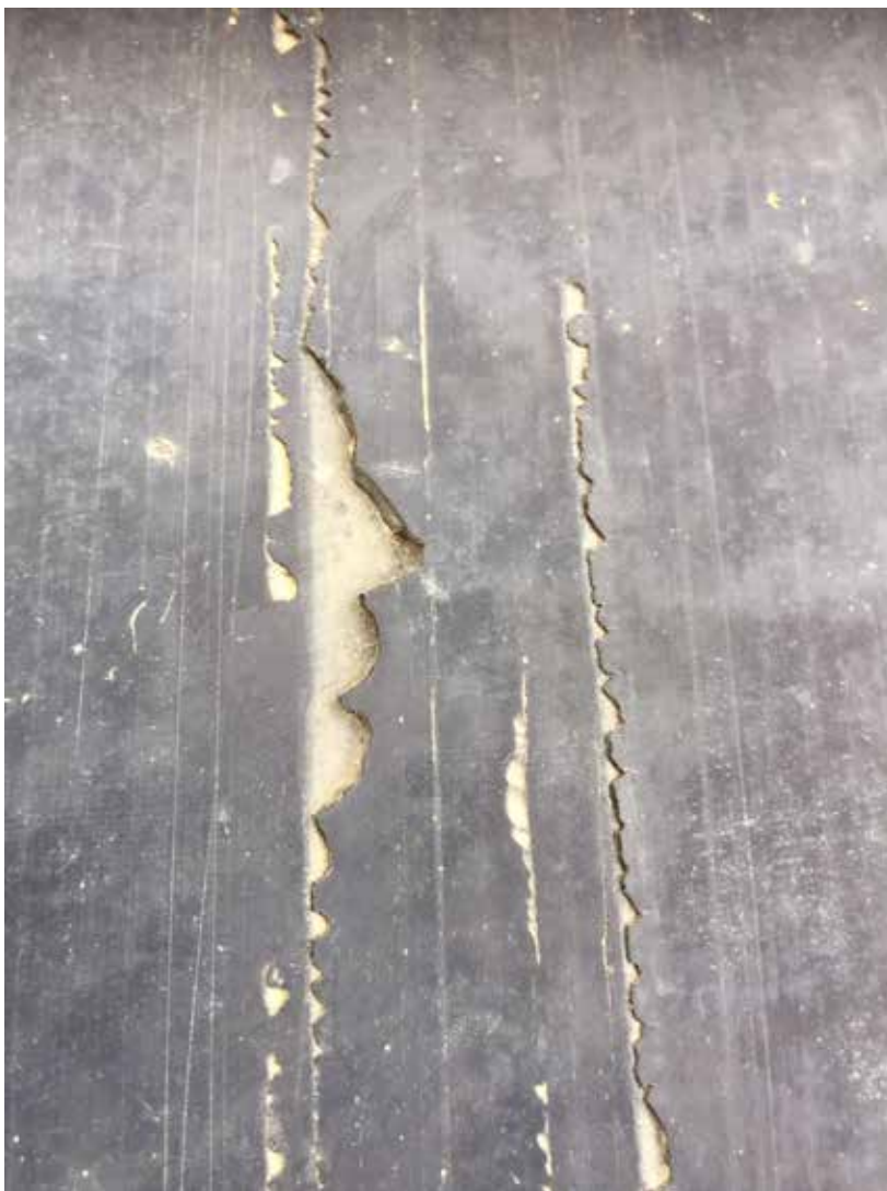
Surface cuts can propagate and link up with other areas of damage, causing pieces of rubber to detach completely if low grade rubber is used.
