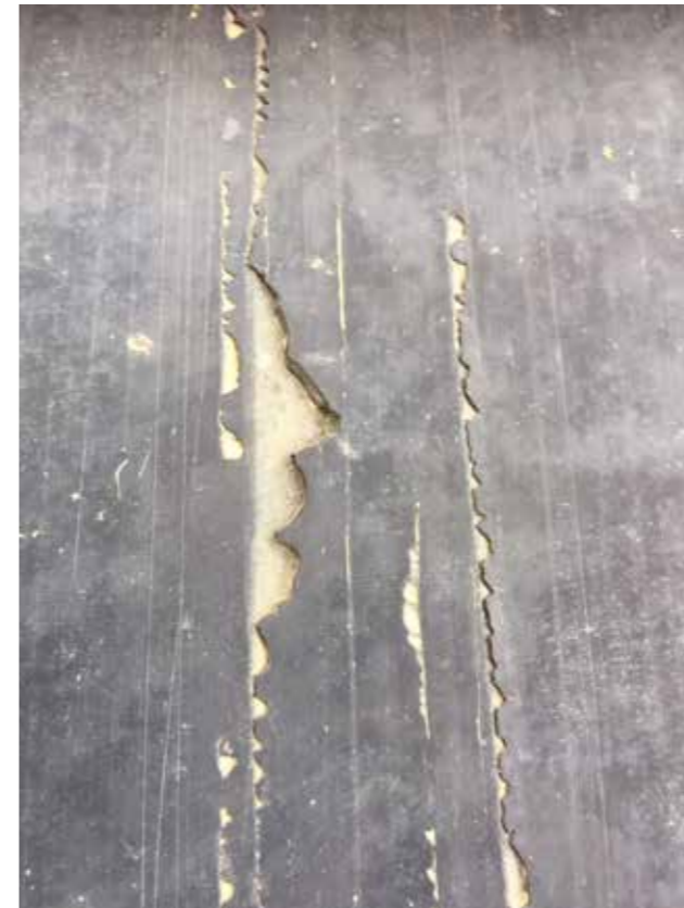
Surface cuts can propagate and link up with other areas of damage, causing pieces of rubber to detach completely if low grade rubber is used.
